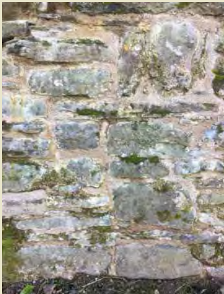
Dividing line between two teams of masons
