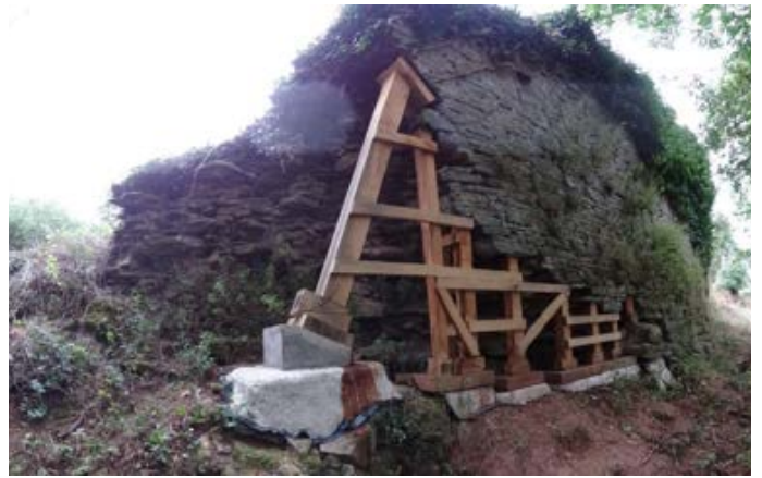
Propped south walls (August 2016)
