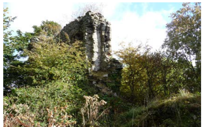
South wall of keep including window embrasure (now being reinstated), 2009
