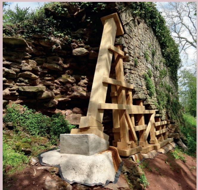
South Curtain wall propping in place
