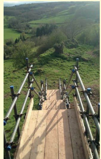
Scaffold staircase April 2016
