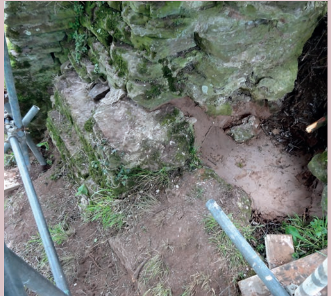
Keep foundations with voids filled in
