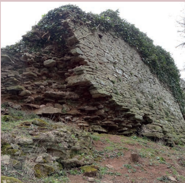
South Curtain walls before propping
