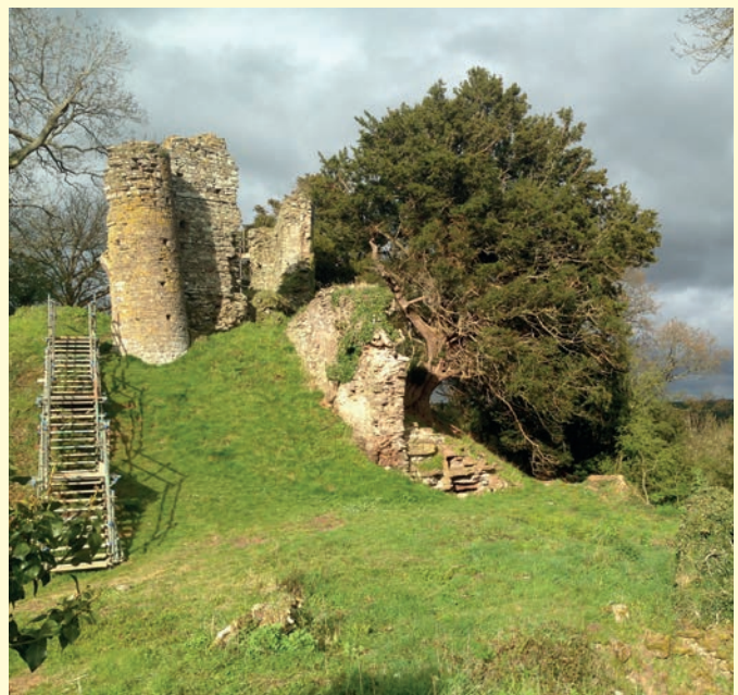
– The first staircase at Snodhill for 400 years
