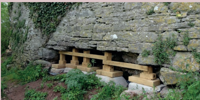
South Curtain wall void propping in place
