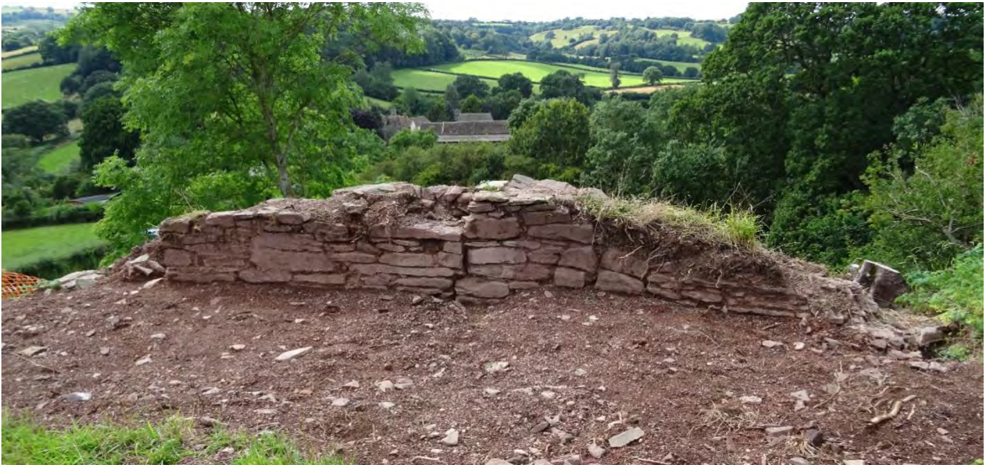
West Fragment with earth pulled back revealing its inside face
