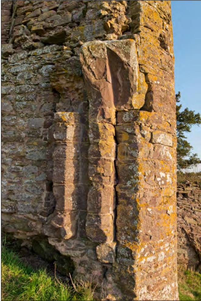
Figure 16 Surviving section of arched head springing from southwest drum tower (DP195801).
