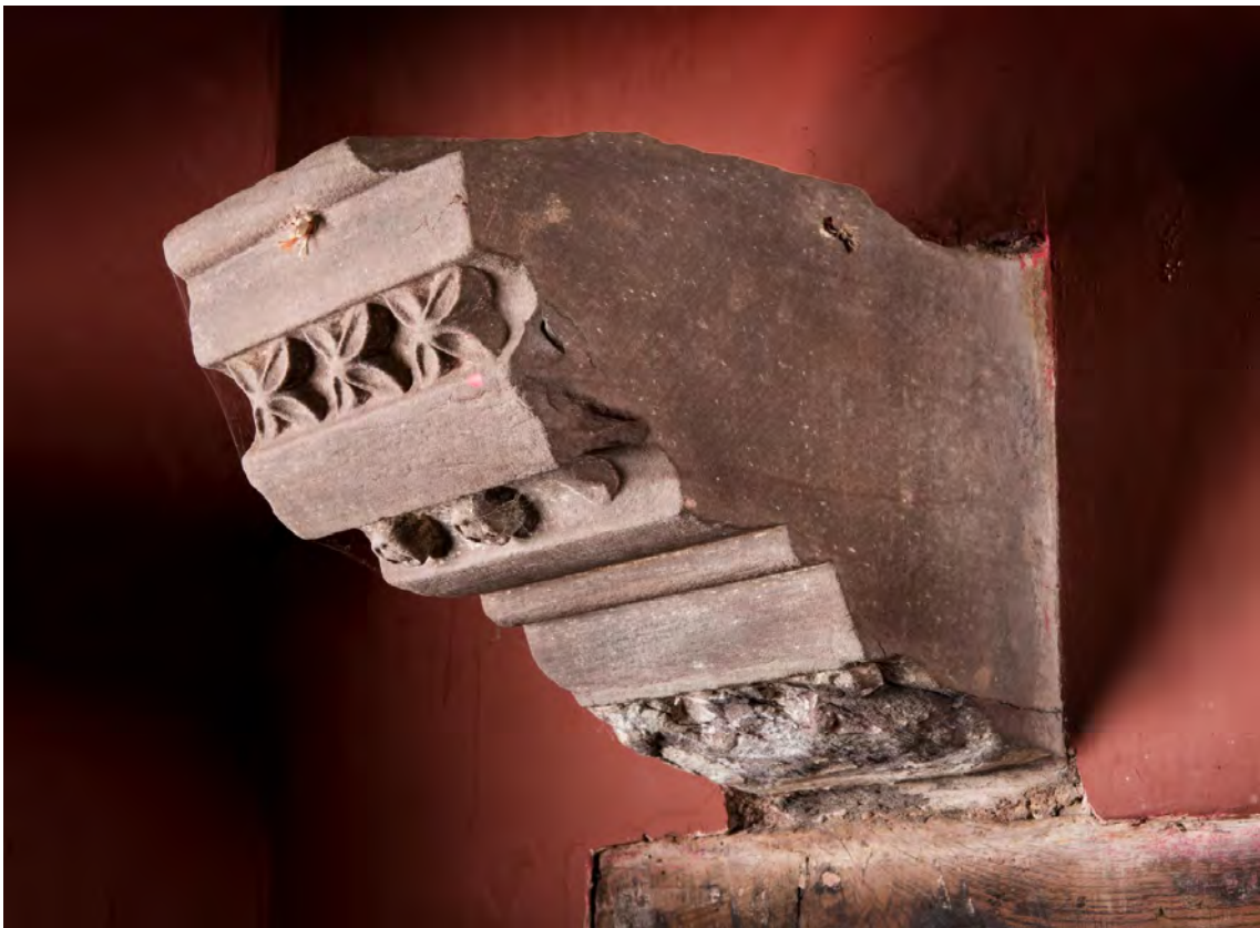
Figure 28 Snodhill Court, corbel over the fireplace in the west elevation of the hall (DP195428).
