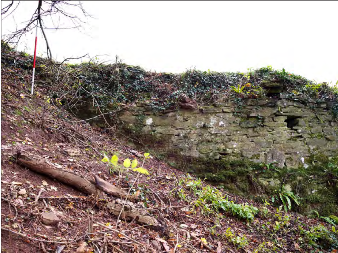
Figure 21 North wing wall, view from south (DP195360).
