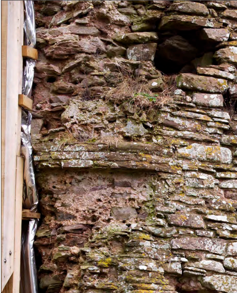
Figure 14 Surviving section of splay for window at the east end of the tower (DP195363 cropped).
