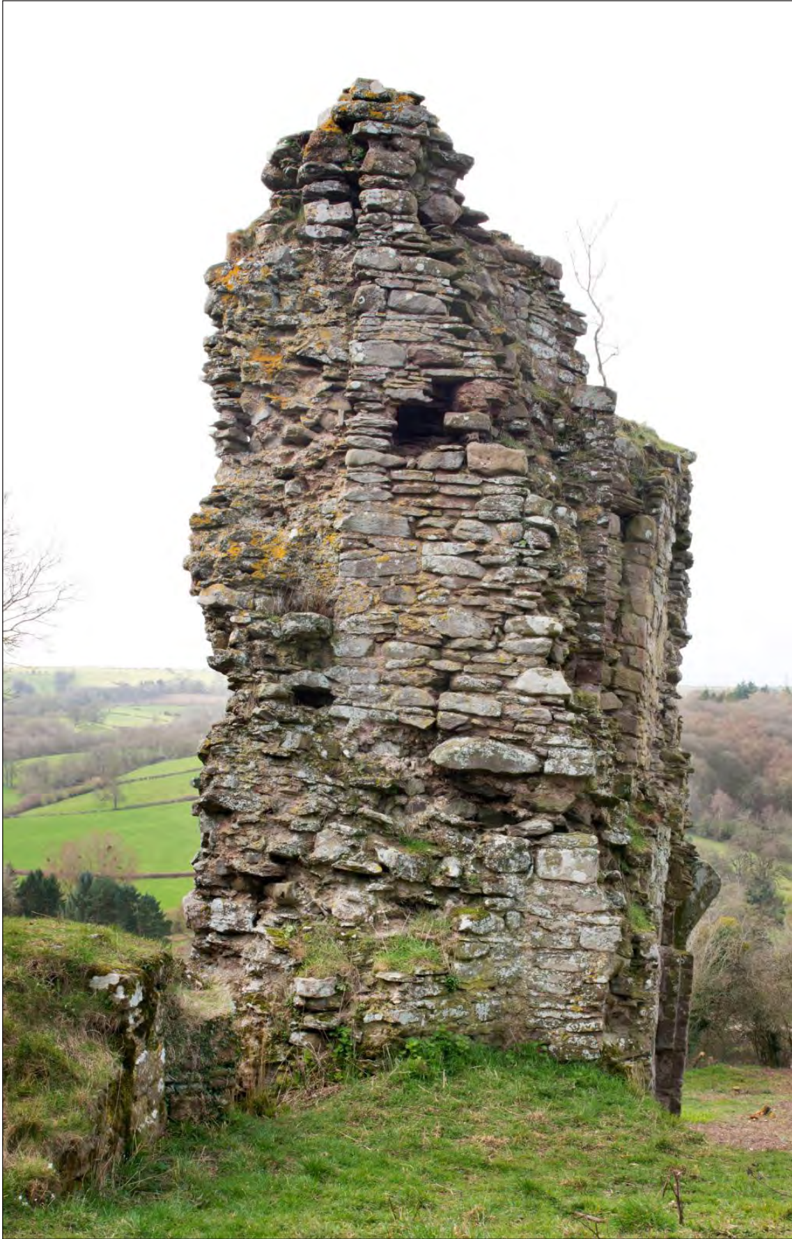
Figure 19 Photograph of the southwest corner of the tower in 2017 (DP195814).
