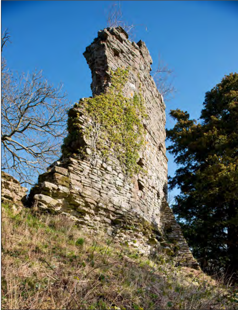
Figure 5 Southeast corner of the tower showing the remains of the plinth at ground floor level (DP195780).
