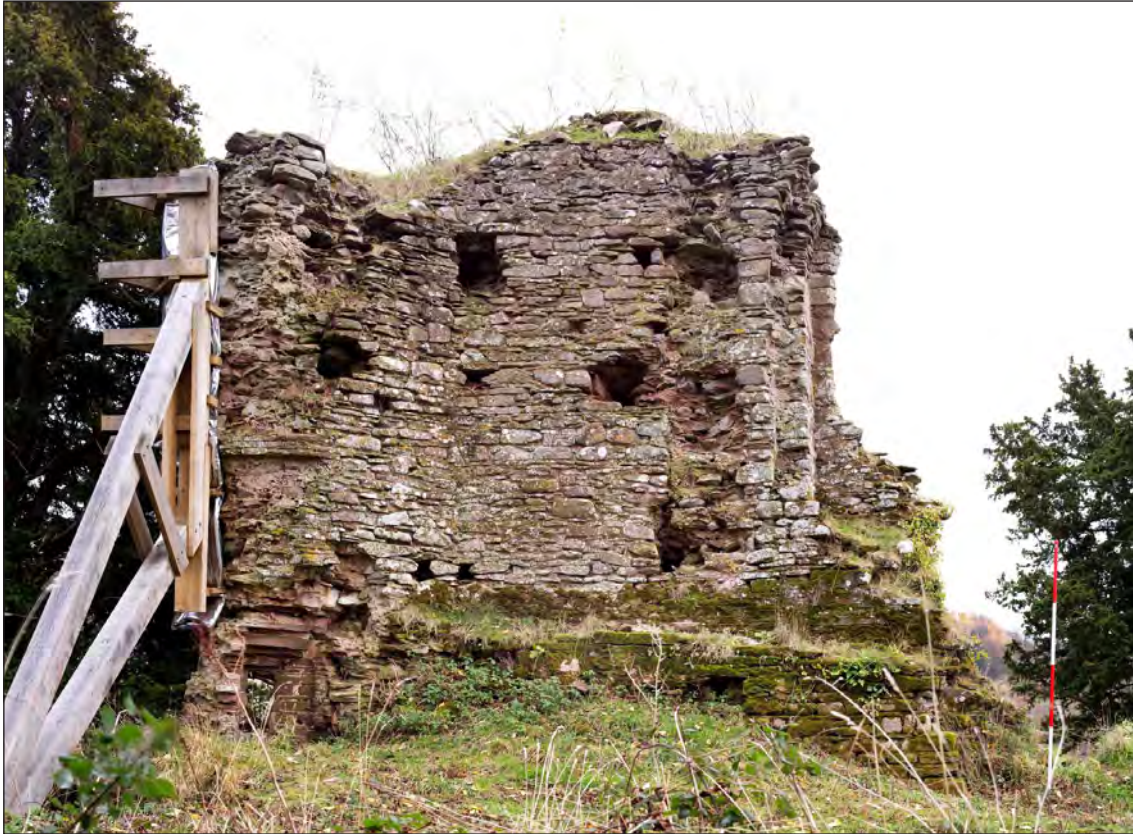
Figure 8 Internal elevation of the south-eastern corner of the tower, showing the offset between ground- and first-floor level (DP195363).
