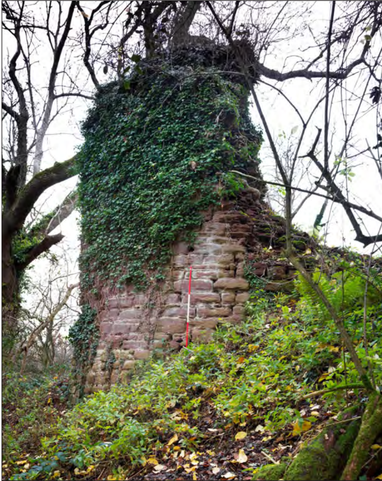
Figure 24 North Tower, view from west (DP195357).
